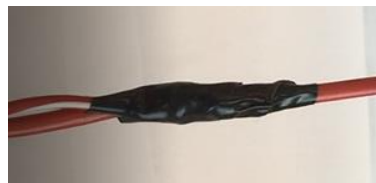
2. Stretch the tape to 3/4 of its original width during application
